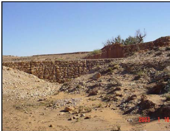
Existing Gabion in Tunisia
